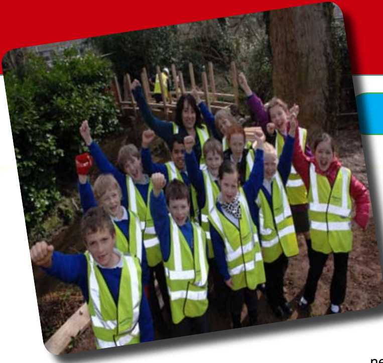
Children from Packington C of E school watching the bridge construction in progress
