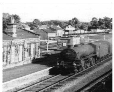
A Class B1 heading a 1959 Manchester bound service as it passes through Quorn & Woodhouse Station. The island platform and goods yard layout design are typical of the GCR
